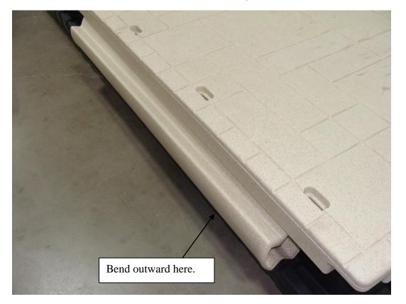
3. Use a mallet and rap along the top and bottom edges of the filler piece so they fit into the channel of the dock section. Filler piece should be flush with the dock edge when finished. Slide the filler piece into the desired location. Tap on the end to move it, if necessary.
