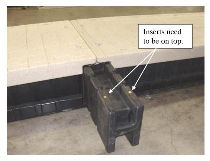
2. Slide the H-Beam all the way into the channel until the inserts align with all four slots on top. The H-Beam should not stick out into the outside channel.
