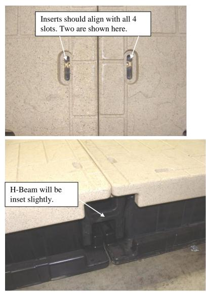
3. Once the inserts are aligned with the slots secure the H-Beam using the  $3/8 \ge 1/2$ " bolts and washers.
